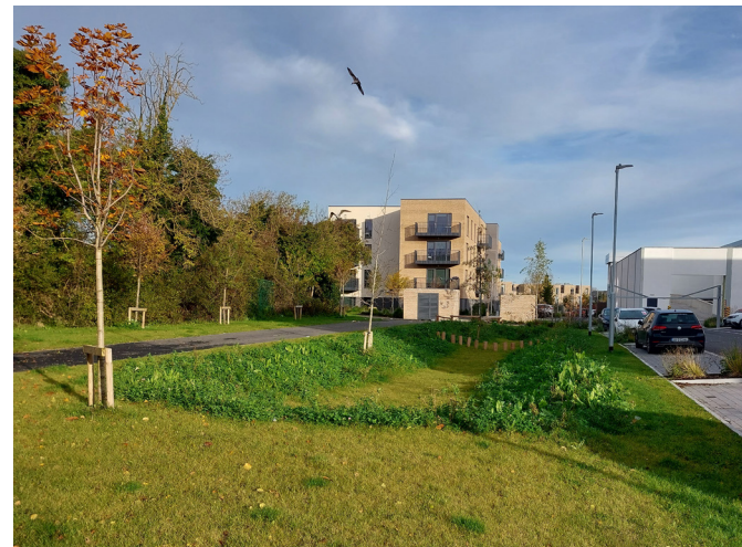
Figure 3-10. INDICATIVE BIOSWALE INTEGRATED IN PUBLIC OPEN SPACE
